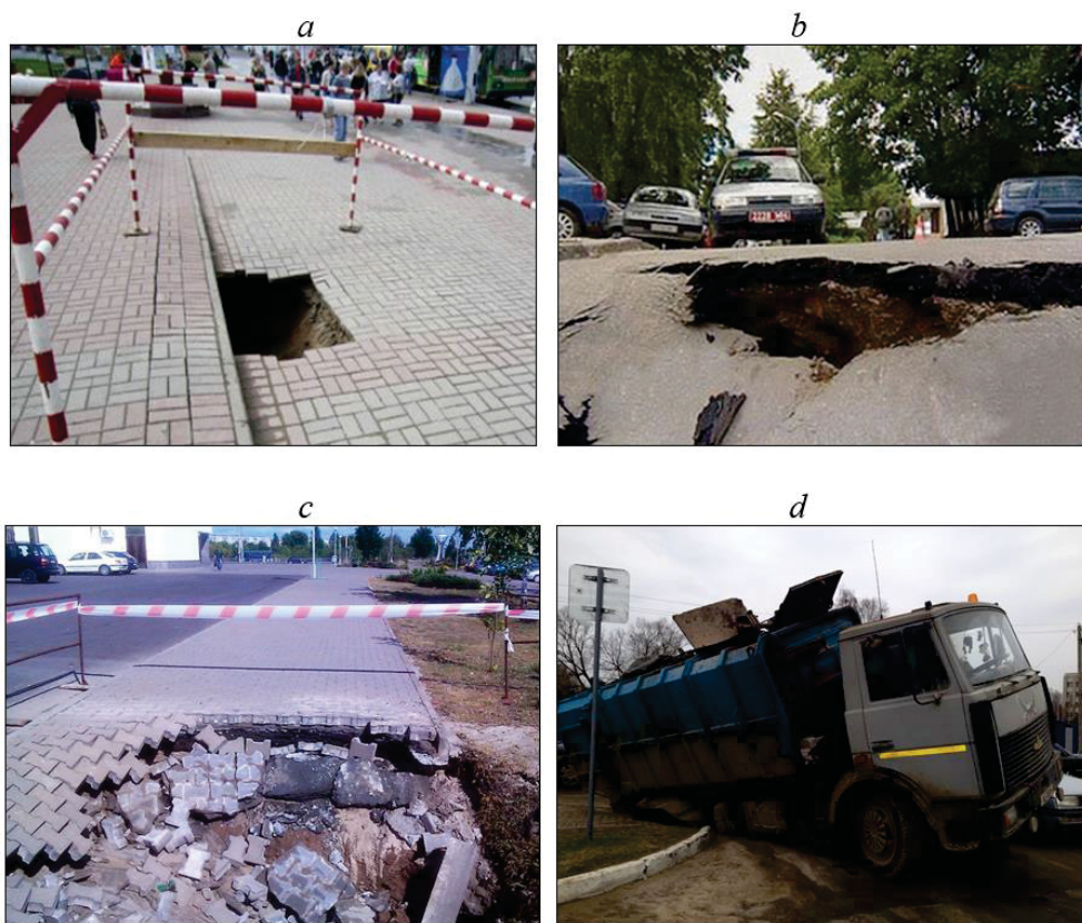
Fig. 8. Deformations of sidewalks and highways caused by suffosion: a) in Vitebsk near the Summer Amphitheater (2012); b) in Minsk along Mogilevskaya street (2014); c) in Gomel near the Ice Palace (2013); d) in Zhlobin near gymnasium no. 1 (2014) [10]
