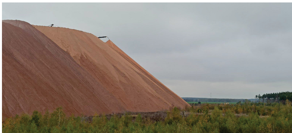
Fig. 6. Transforming of the natural surface topography: a ) phosphogypsum dumps of the Gomel chemical plant (October 2020); b ) salt dumps of the JSC «Belaruskali» (October 2020). Photo by O.V. Shershnev
