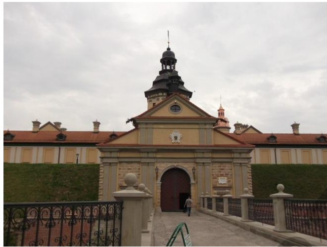
Figure.90. Slutskaya entrance gate of Nesvizh.
