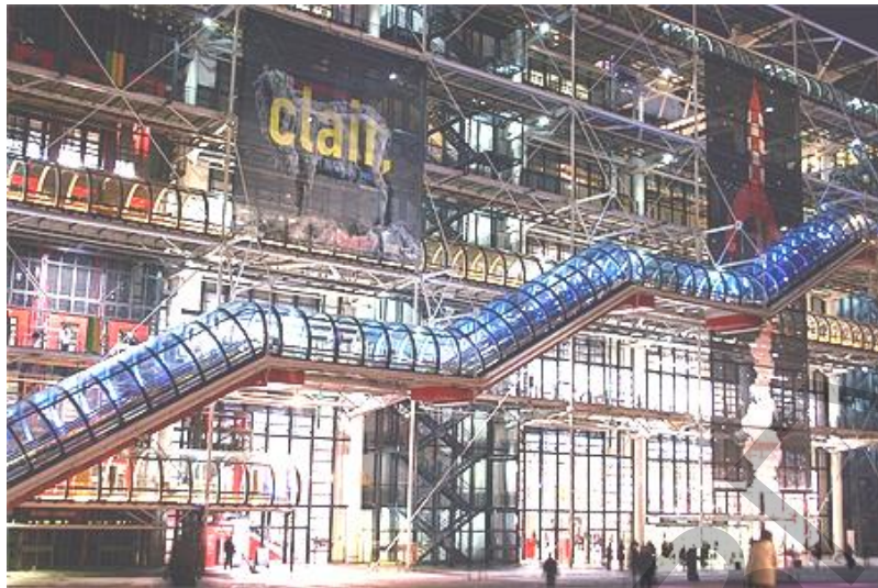
Fig. 69. Centre Pompidou arts, Architects r. Piano and r. Rogers. 1986 year.
