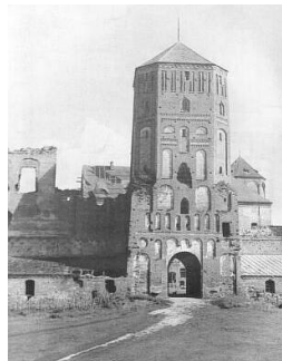
Figure. 107. Even in Soviet times, architects were thinking how to deal with these ancient stones. Some have suggested simply bulldoze them with the Earth.
