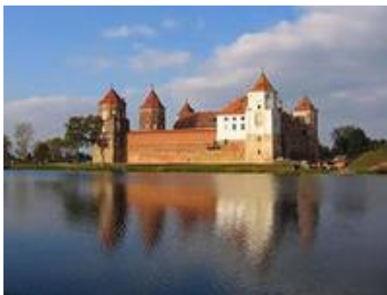
Figure. 84. The Mir castle is an architectural historical ensemble. The contemporary condition.
